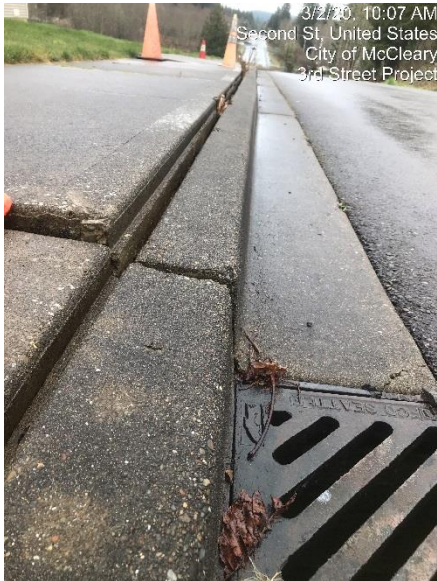
#1- Tree Root Damage on sidewalk installed in 2007.
