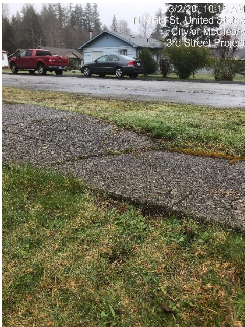
#2- Damage from vehicle on sidewalk. Installation unknown.
