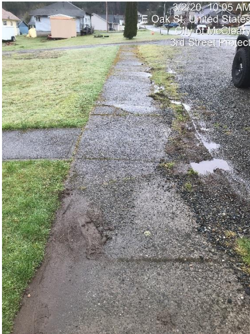
#3- Vehicle Damage on sidewalk. Unknown installation
