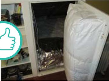
**WEATHERSTRIPPED AND INSULATED HATCH**
