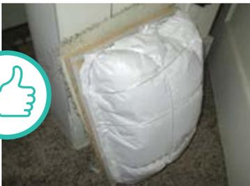
**CRAWL HATCH INSULATED AND WEATHERSTRIPPED**
