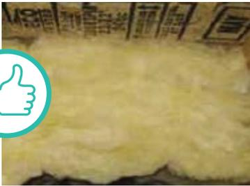
**INSULATION IN FULL CONTACT WITH FLOOR**
