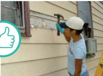
**INSULATION ACCESS HOLES PLUGGED AND SEALED WITH SOLID PLUGS**
