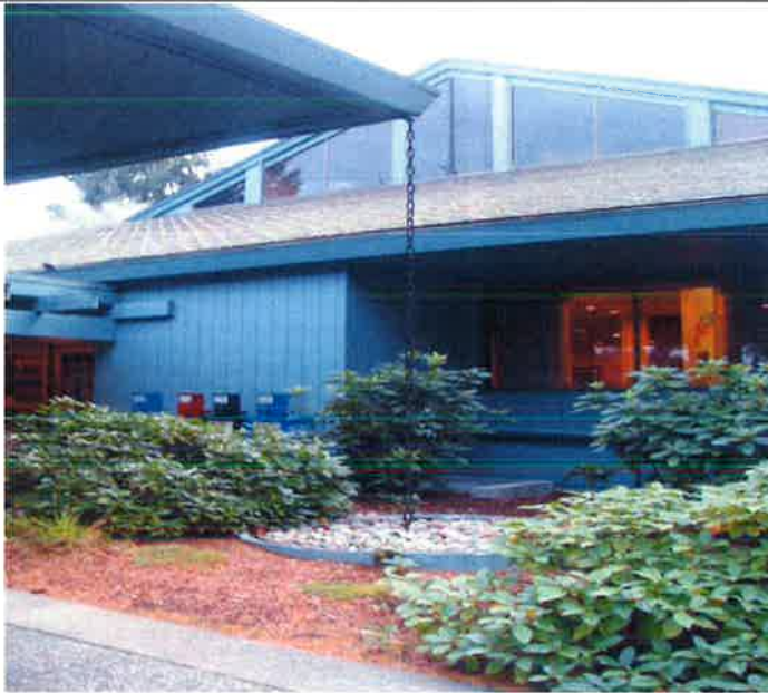
Infiltration and recharge of roof runoff into stone infiltration chambers via “rain chains”
